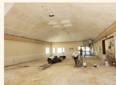
Parish Hall Remodel 3
