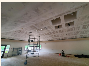
Parish Hall Remodel 2
