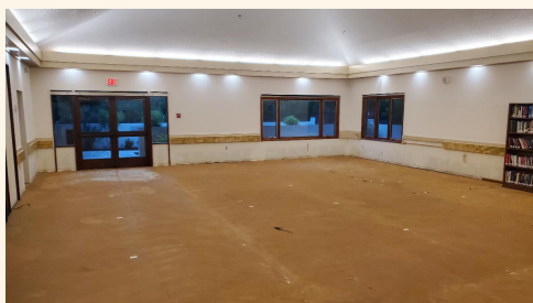
Parish Hall Remodel 1
